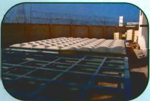
Steel Flooring for GRP Tank
