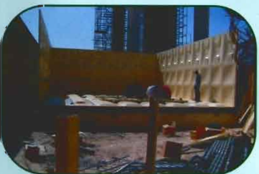
Technicians working on base of GRP Tank
