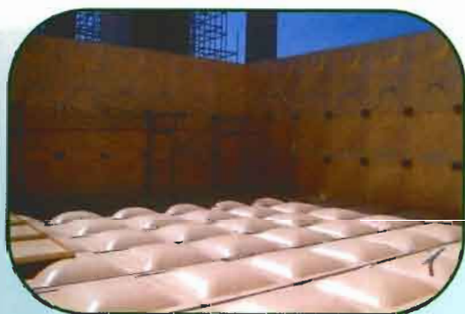
Bottom & side panel erection completed
